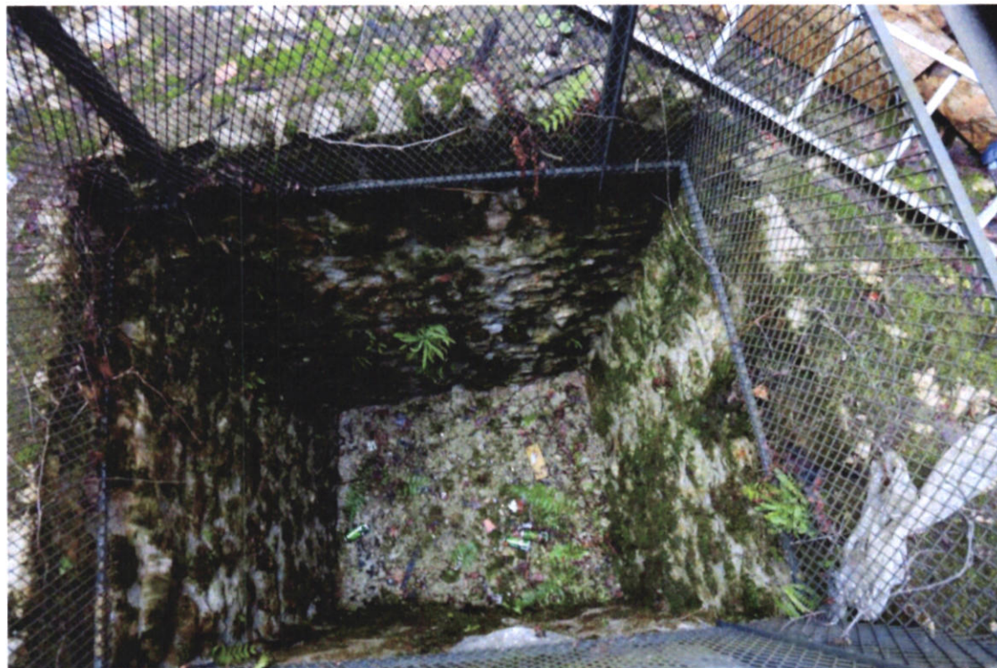
Cisterna (C I)
