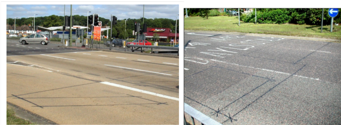
Figura 44 – Bucle inductive instalate in asfalt (exemplu)
