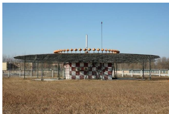
Figure 8: DVOR Site typical structure
